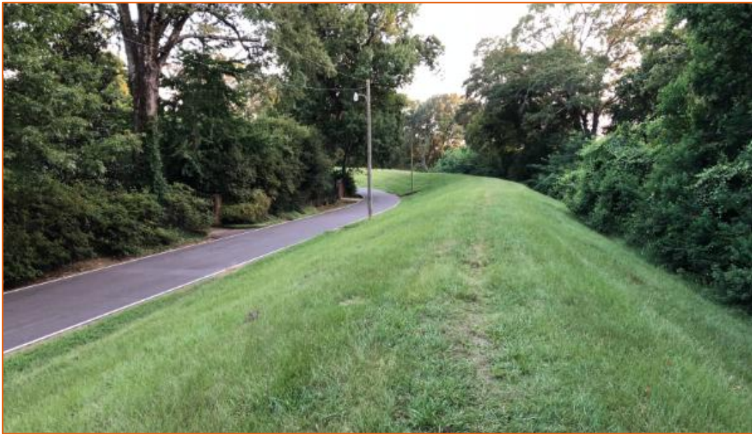
Figure 1-6: Example Levee Embankment supporting recreational pathway.
