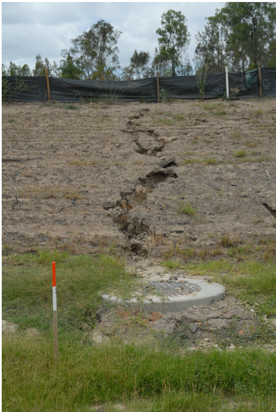
Figure 5.1.4 Batter erosion to dispersive subsoils
