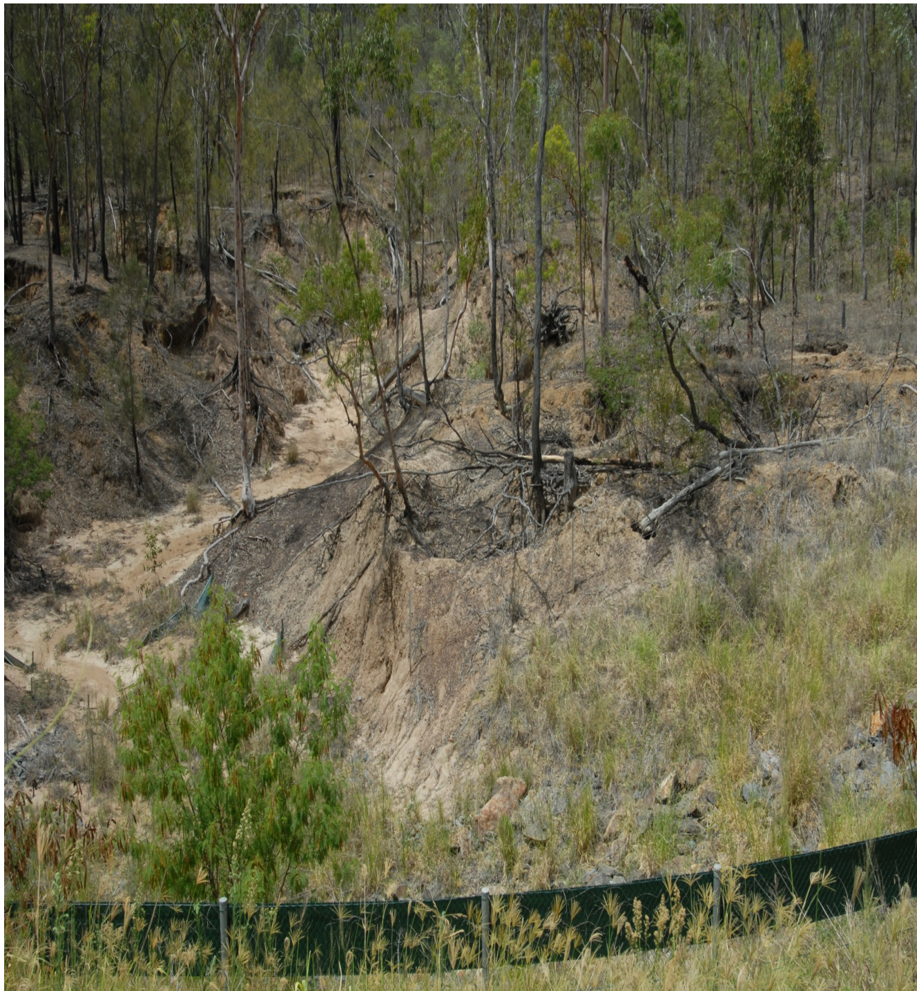
Figure 5.1.3 Erosion and dispersion along service trench
