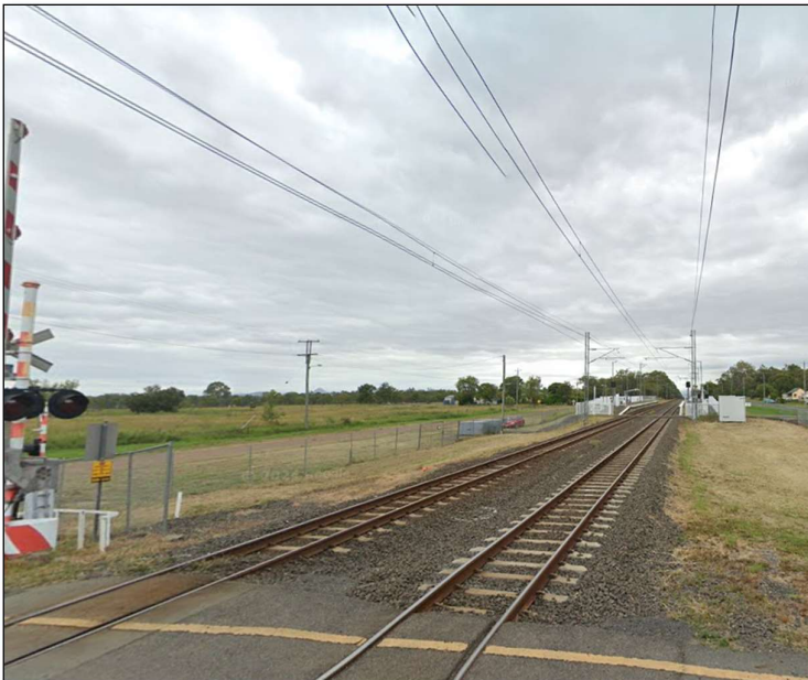
Figure 3: Thagoona Train Station
