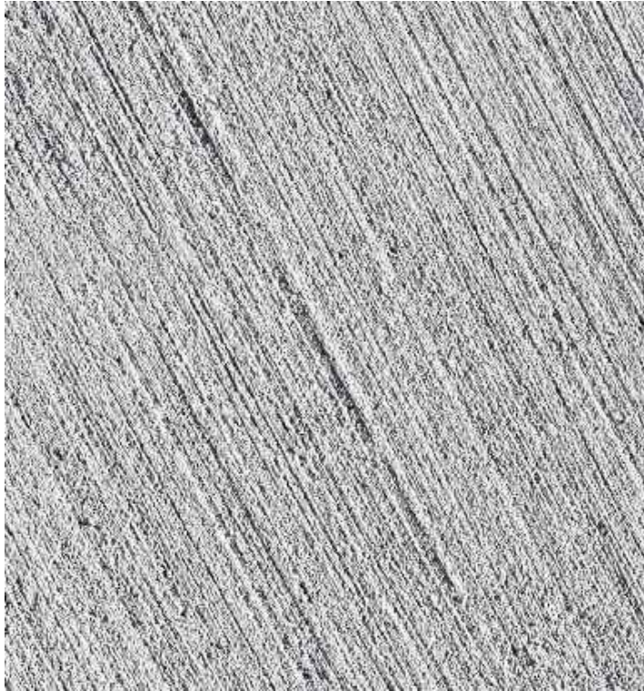
Broom Finished Concrete (varying directions)
