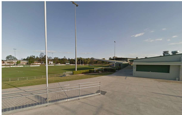
Figure 4: Existing western grandstand (Source: Google Maps, 2026)
