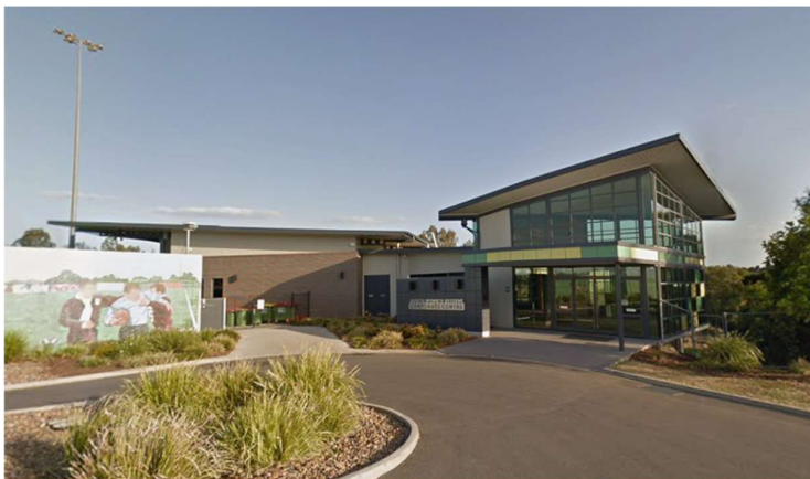
Figure 5: Existing corporate centre (Source: Google Maps, 2026)
