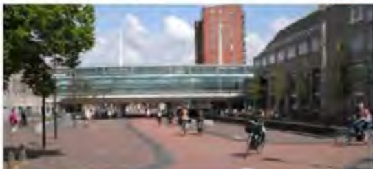
Houten Station, Houten (Netherlands) 100% of space for pedestrians and cyclists
