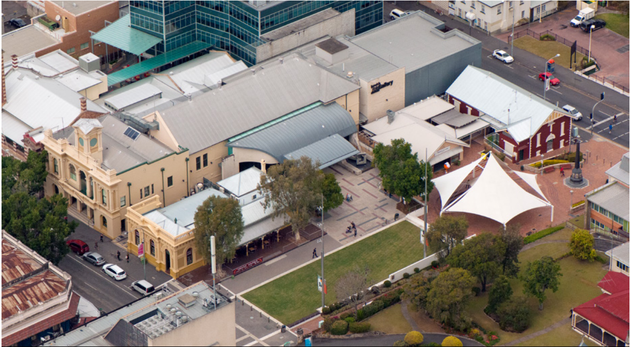
d'Arcy Doyle Place (Art Gallery Forecourt) – 116 Brisbane Street, Ipswich
